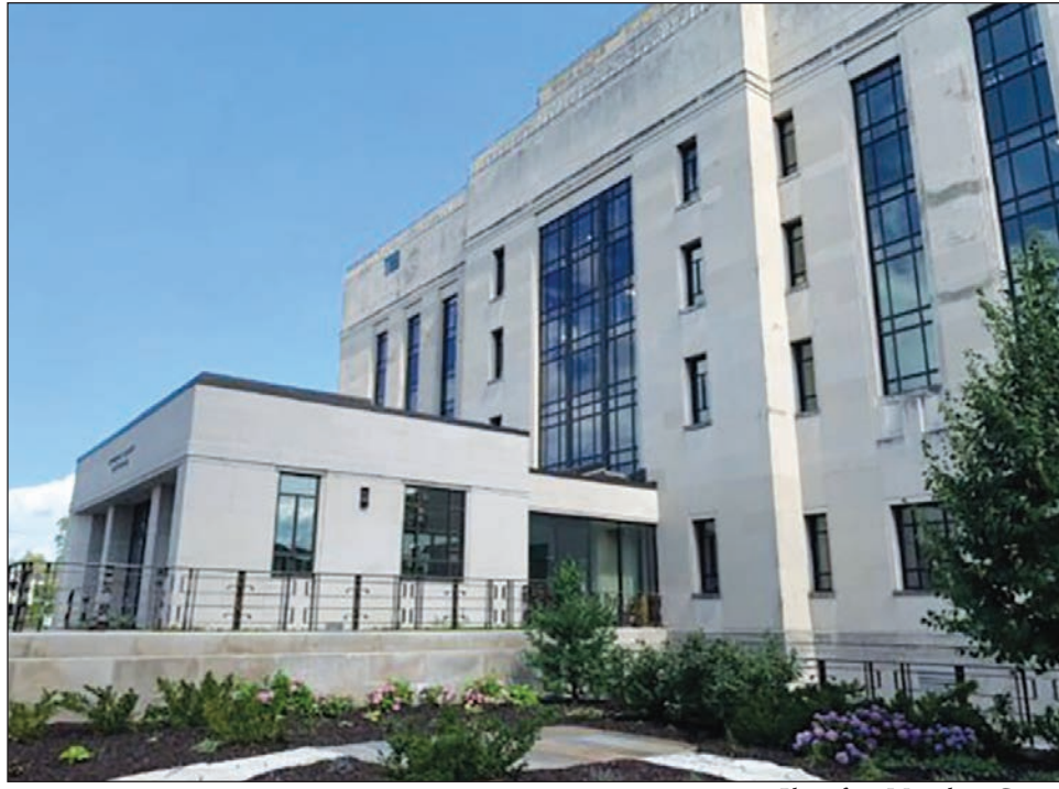
The courthouse in Oshkosh is one of the county buildings that is considered to have challenges, as it does not meet current standards for maintaining safety in a court facility.
