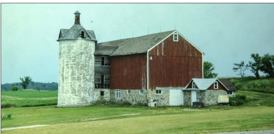
A silo with a unique and beautiful roof.
