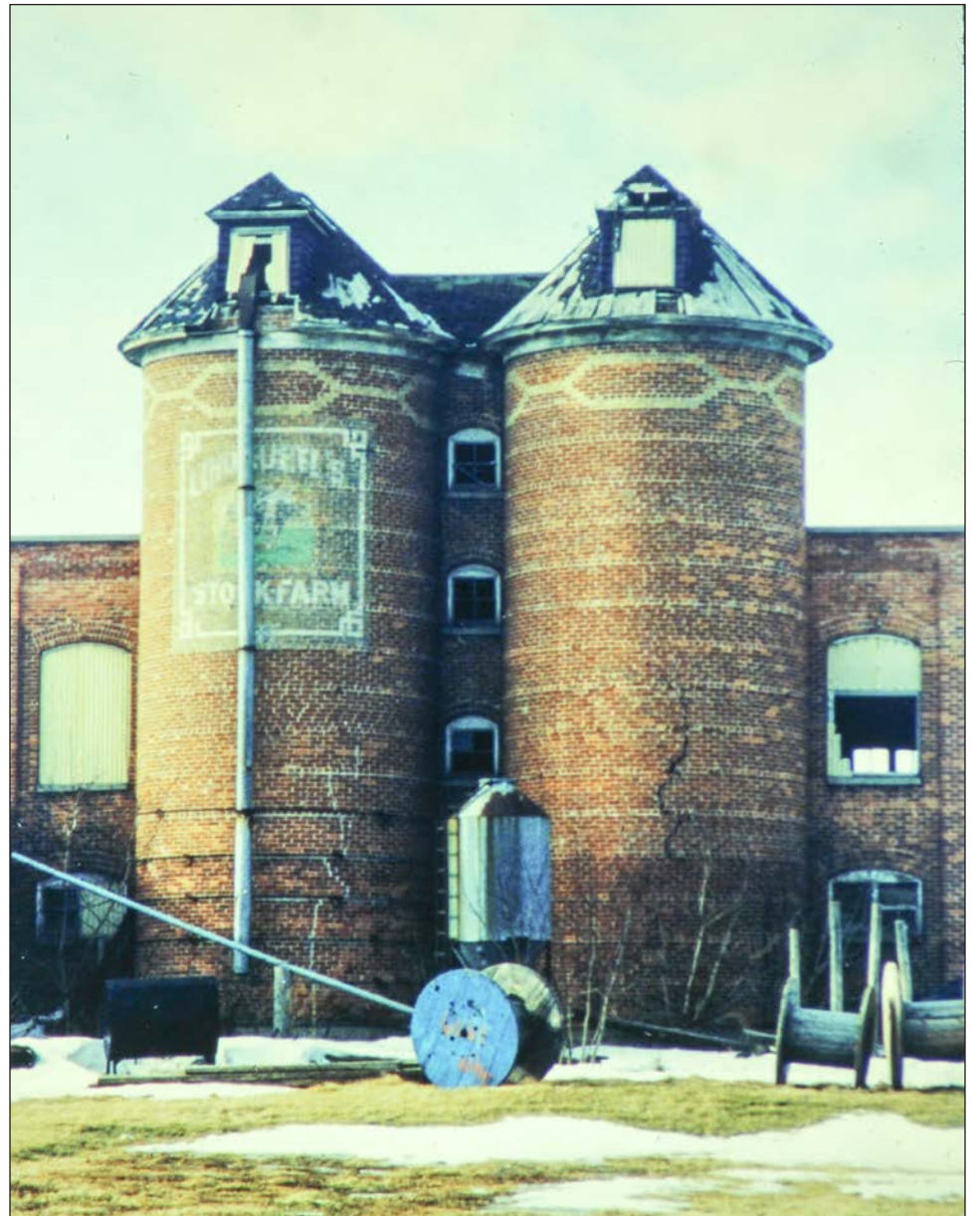
Twin silos located in Door County, WI.
