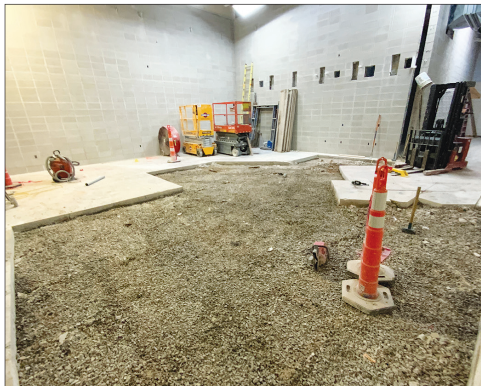
Progress continues on the building's maintenance area.
